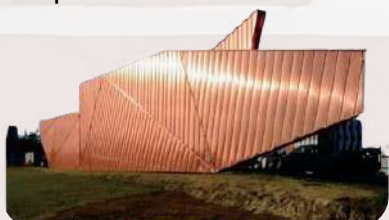
Copper / Bronze / Zinc Façade
