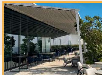
Fabric Retractable Roof
