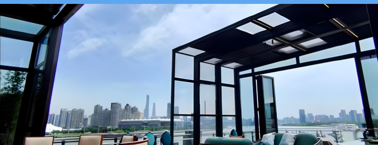
Restaurant Roof and Mall Roof
